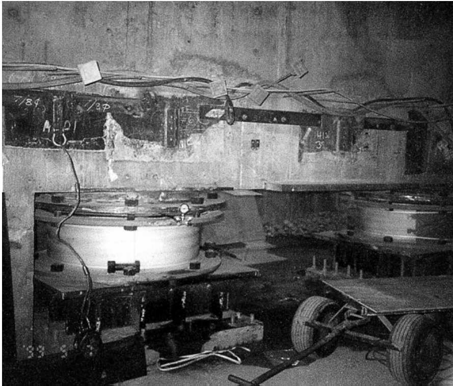
Figure 17. Photograph of HDR bearings installed under tower walls
