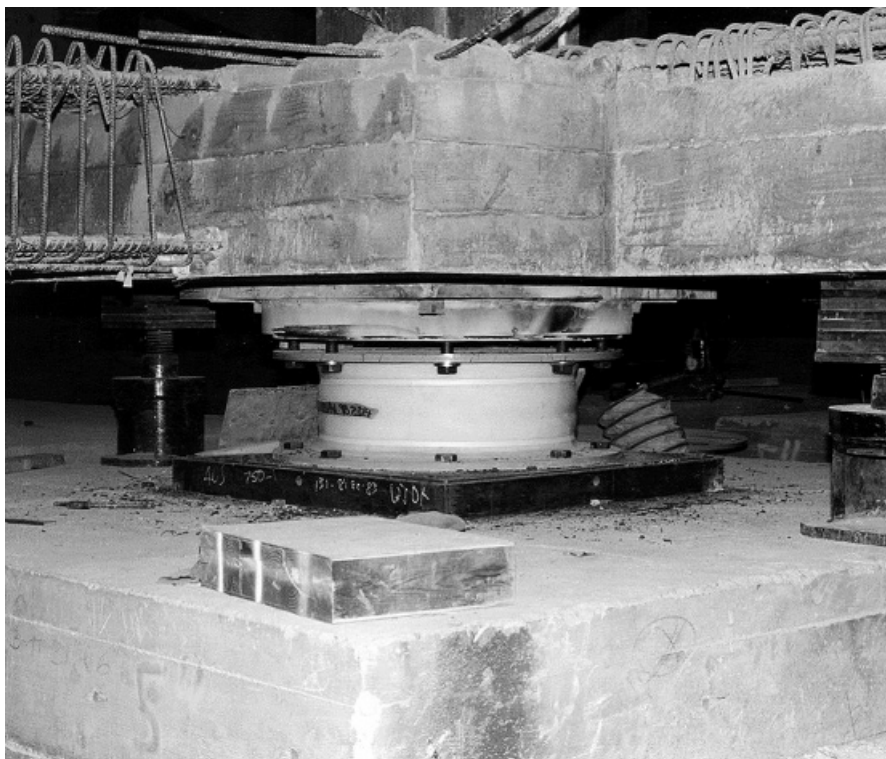
Figure 18. Photograph of HDR bearing installed under stand-alone column
