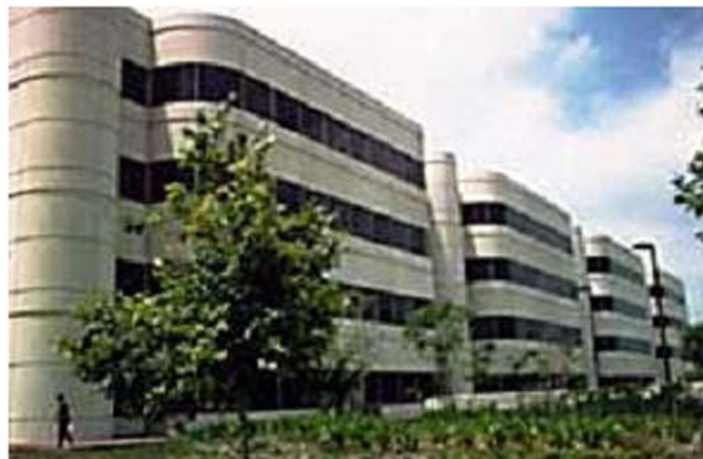
FIGURE 8 The Foothill Communities Law and Justice Center (FCLJC), completed in 1985 in Southern California, is the first base-isolated building to be built in the United States. Courtesy of James M. Kelly with permission [Colour figure can be viewed at wileyonlinelibrary.com ]
