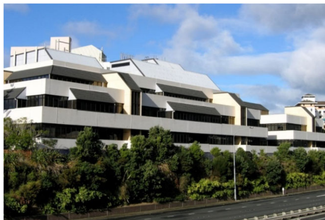
FIGURE 4 The William Clayton Building, completed in 1981 in New Zealand, is the first base-isolated building to be built on lead-rubber isolators [Colour figure can be viewed at wileyonlinelibrary.com ]
