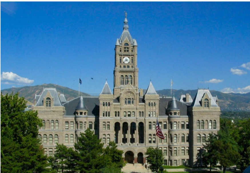
FIGURE 9 The Salt Lake City and County Building is the first historic building in the USA to be seismic retrofitted with seismic isolation. A total of 447 lead rubber bearings were instead on top of the original strip footings of the building with a new concrete structural system built above the isolation bearings 61 [Colour figure can be viewed at wileyonlinelibrary.com ]
