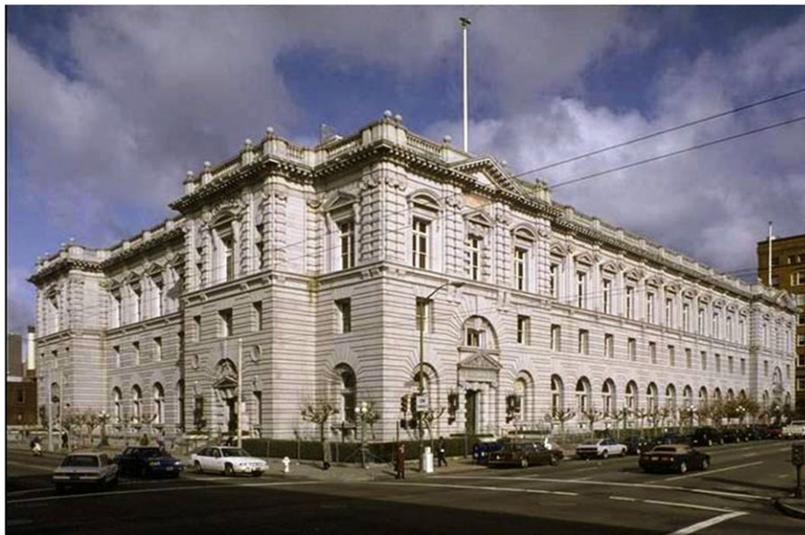
FIGURE 13 The US Court of Appeals in San Francisco, California is the first building in the USA to be isolated on a single concave, sliding isolation system in 1993. Courtesy of Michael C. Constantinou with permission [Colour figure can be viewed at wileyonlinelibrary.com ]
