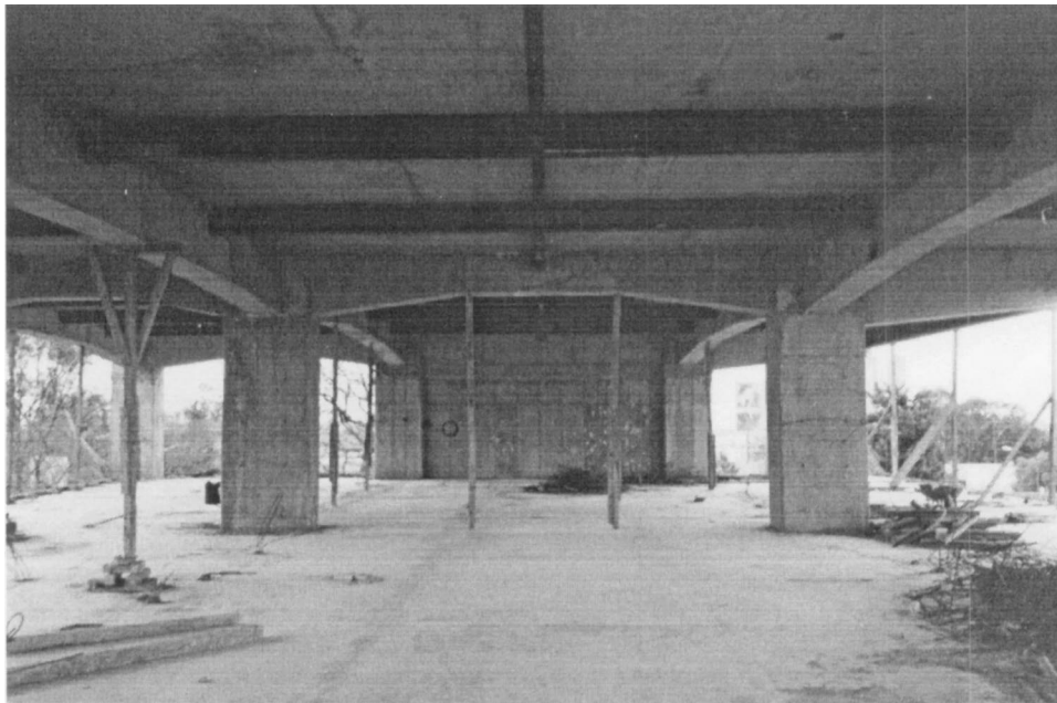
Fig. 1. Building with RC haunched beams currently under construction in Mexico City
